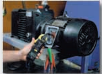
Testing repaired pump
