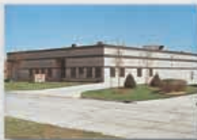
Factory Service Center - Illinois Phone 630-545-1310
