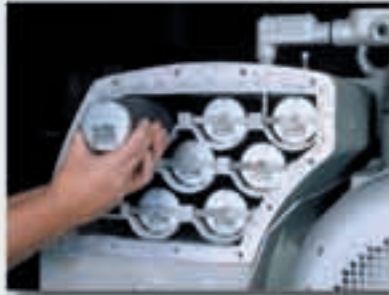
Installing exhaust filters in R5 pump
